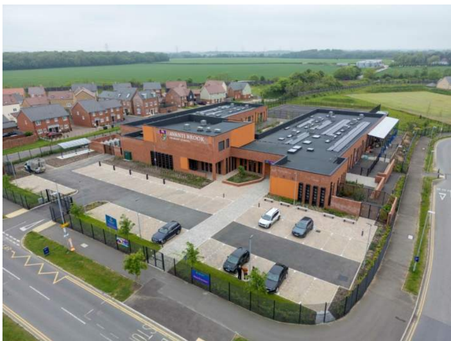
Timber Frame / SIPs Construction – Avanti Brook Primary School, Bishop's Stortford
